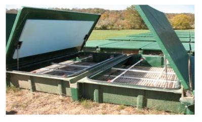
AdvanTex System -Recirculating packed bed filter that uses a highly absorbent engineered textile for the treatment media
